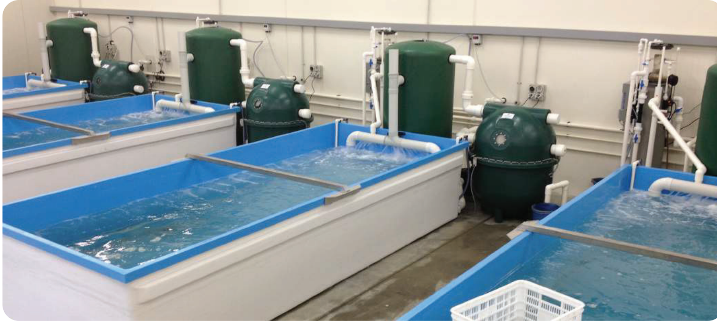
PG filters in an aquaculture facility
